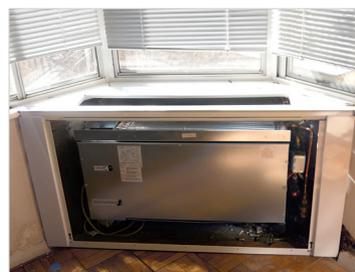
*The custom-built enclosure consisted of the top, two legs, base and front covers.*
