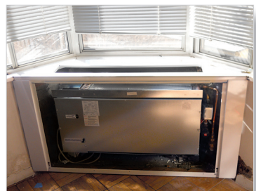
The custom-built enclosure consisted of the top, two legs, base and front covers.
